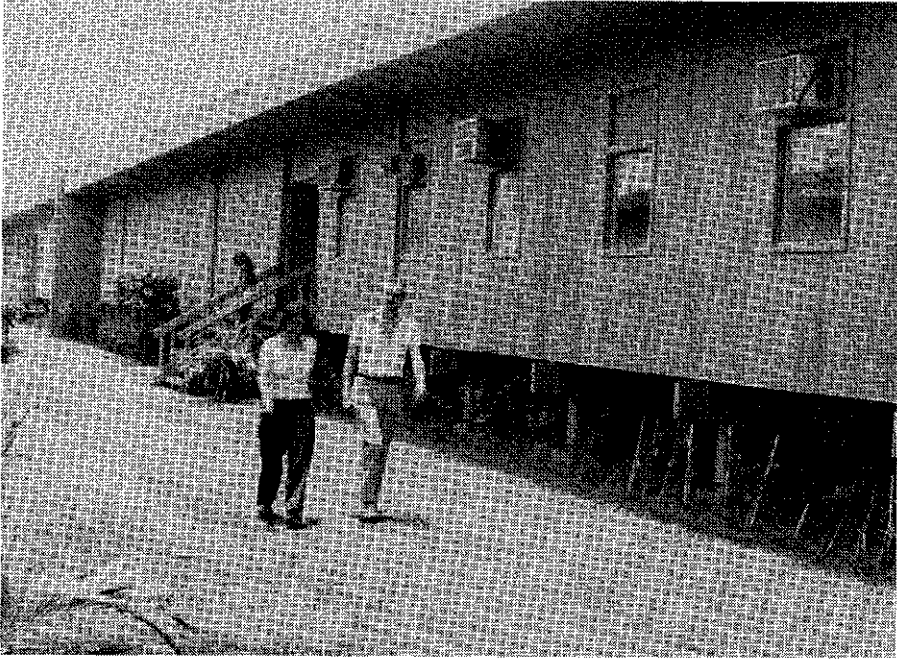
Temporary classroom buildings at the 'Quarry'
